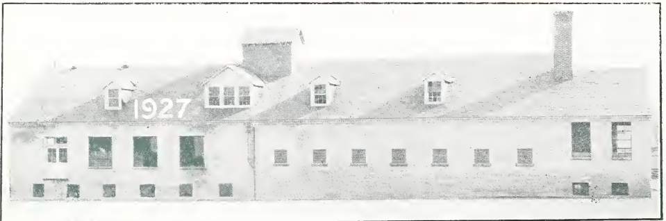
The New Seed-Corn Drying-Plant—Erected in 1927.
